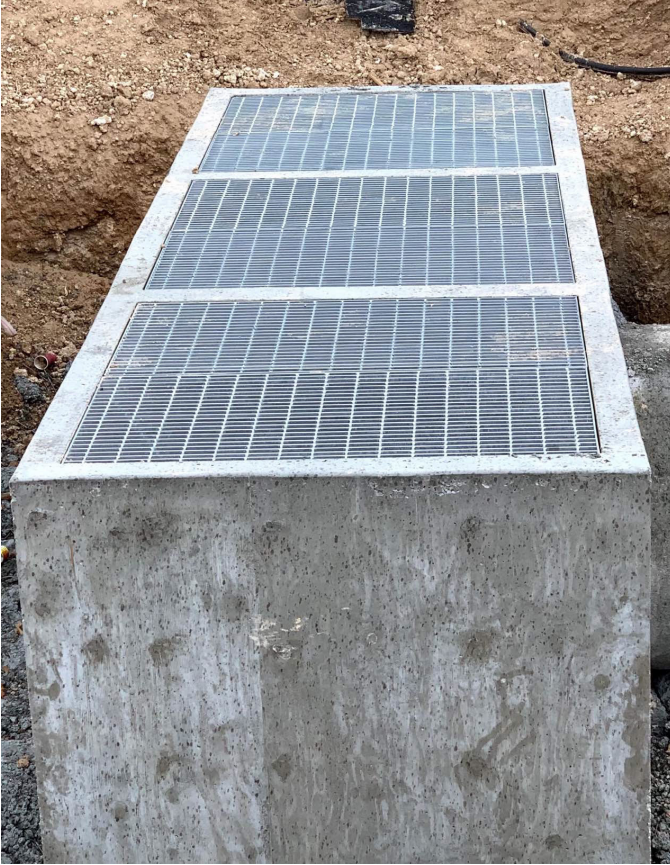
Grate in Concrete
